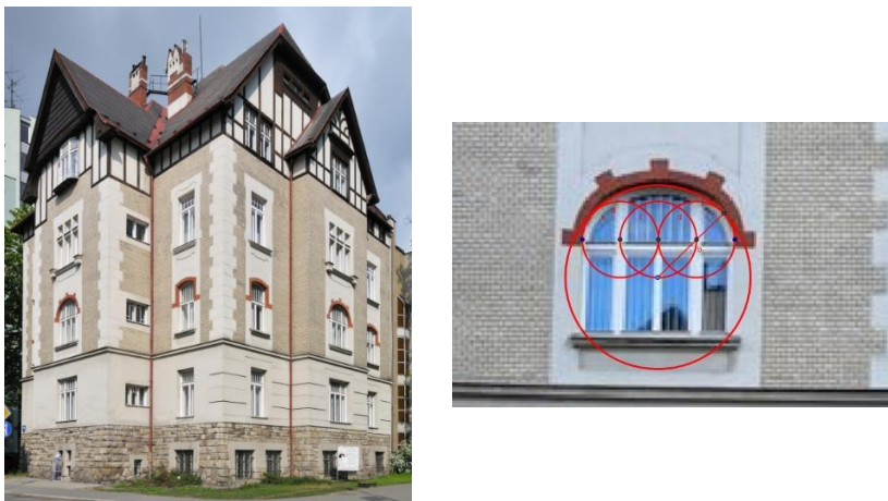
Fig. 6: Building and its detail on Milíčova Street, Ostrava
