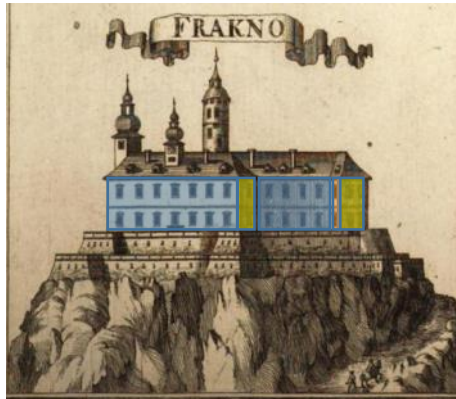
Fig. 2: Vertical orthogonal projection on the veduta of Frakno Castle created by Justus van der Nypoort [1]
