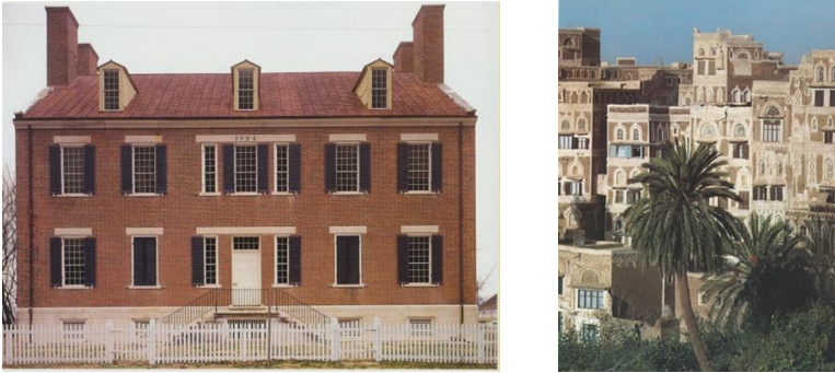
Fig. 6: Examples of multilevel mirror symmetry of facades and its details. Left: Shaker's house (USA), ([5, p.56]); right: Shibam houses (Jemen).
